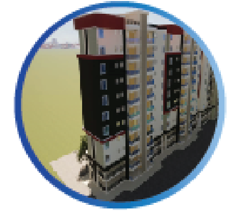
Completion In 24 Months
